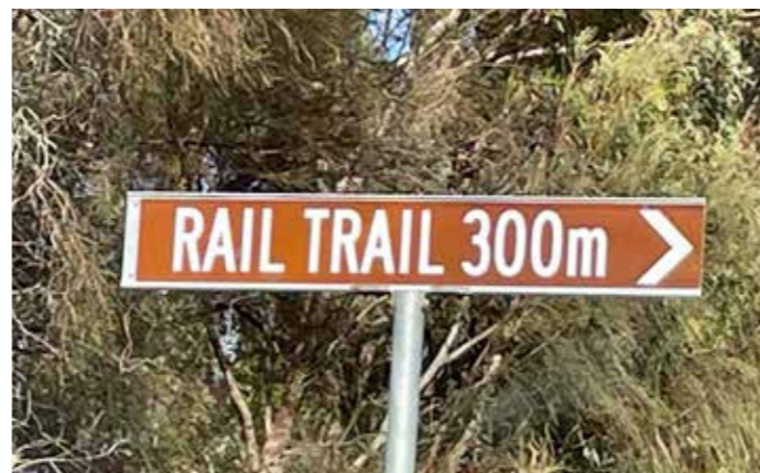
Grampians Rail Trail - Wrong sign type, this sign suggests that the rail trail is 300m off the road, not 300m up the road
