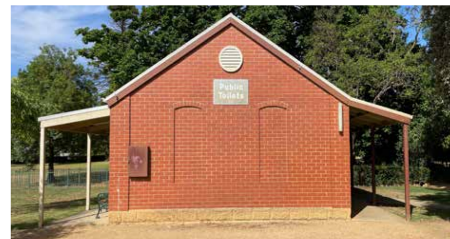
St Arnaud - Queen Mary Botanic Gardens public toilets - This wall with a shelter roof would make an excellent location for a visitor information board.
