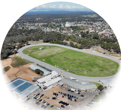
Lord Nelson Park Precinct Sports Lighting and Oval Resurfacing
