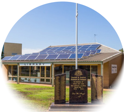
Stawell Library Refurbishment
