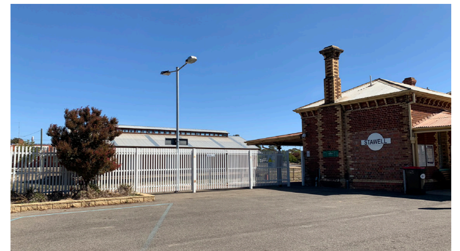
Stawell Train Station
