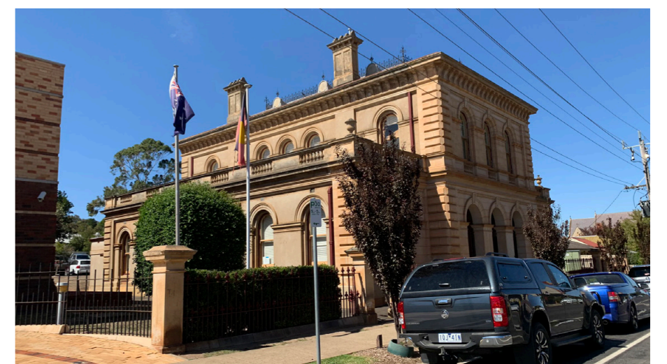
The VHR building in Patrick Street
