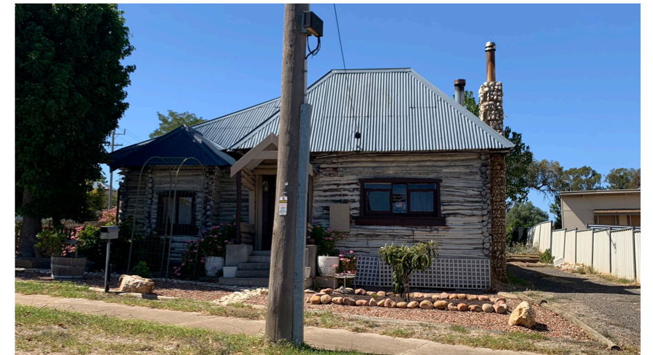
Detached, single storey dwellings are typical of the residential areas
