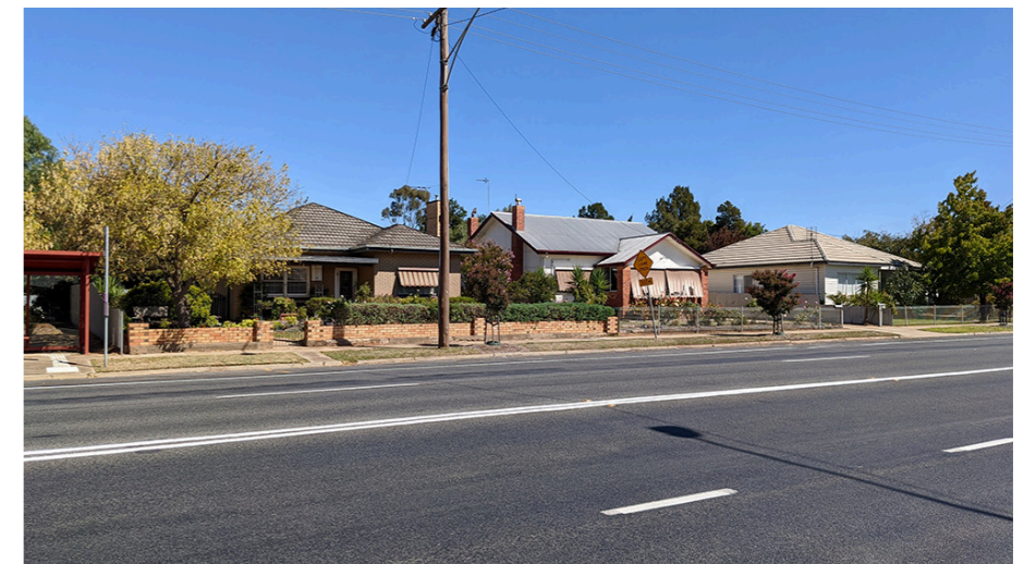
Residential building fabric toward the north of the study area
