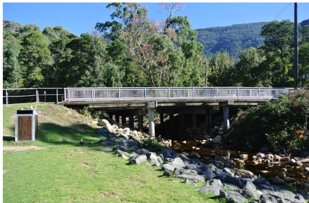
Figure 22. Existing Stoney Creek bridge
