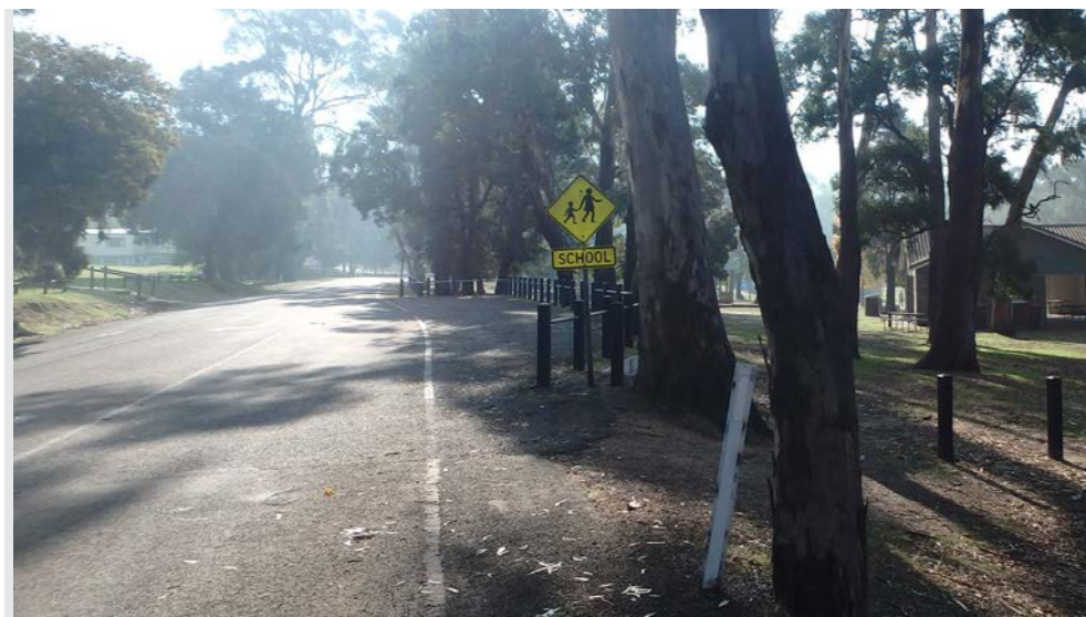
Figure 34. Existing conditions of Grampians & School Roads junction
